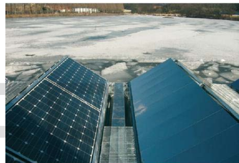
Fig. 10. 20kWp FTCC System in Cheogji, South Korea with can withstand water freezing temperatures [24]
