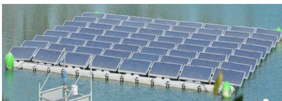
Fig. 9. 14kWp Floating System in Piolenc, France [21]
